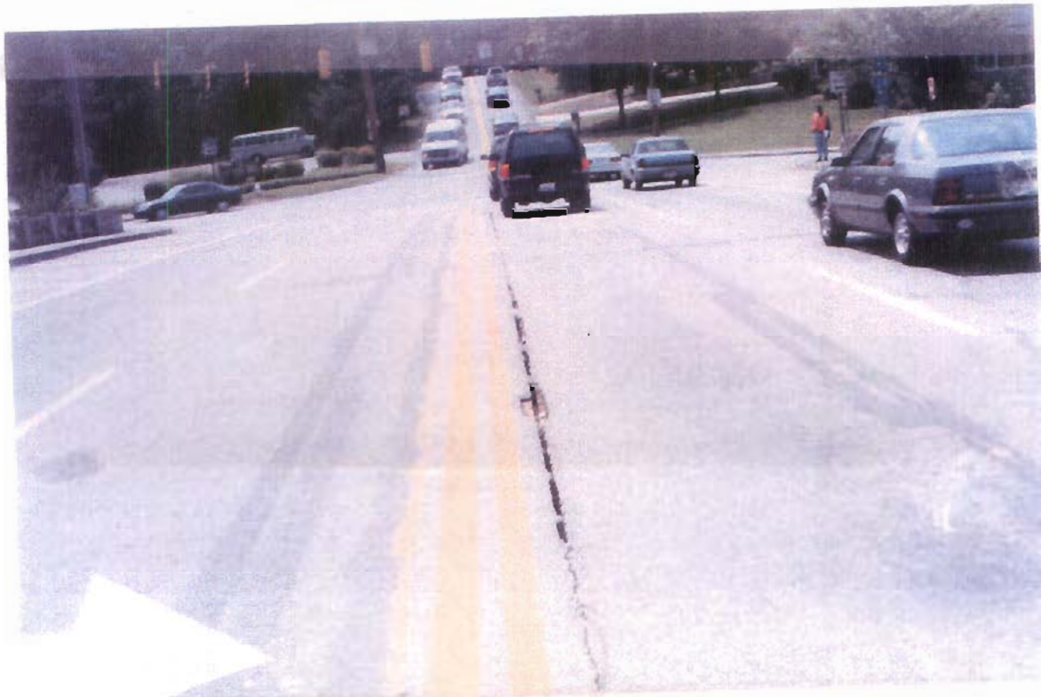
LARGE CRACK ALONG CENTER LINE
