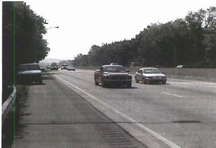
LOOKING AHEAD ON UNDERPASS ROUTE
