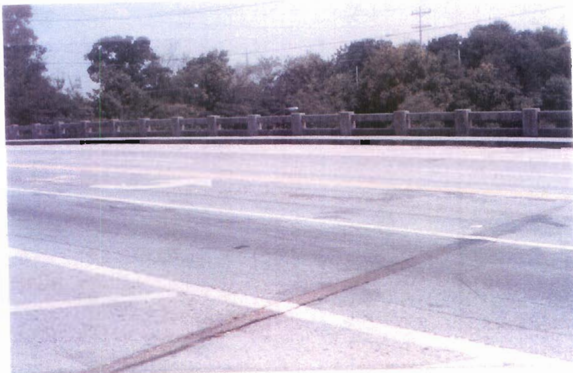
LARGE CRACK ALONG CENTER LINE
