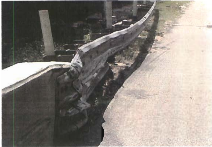
DAMAGE GUARDRAIL
